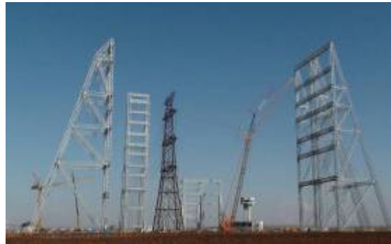
UHV engineering test center
