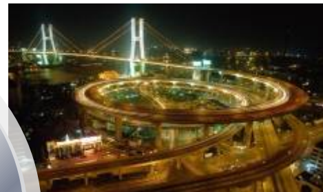
Ensuring power supply
