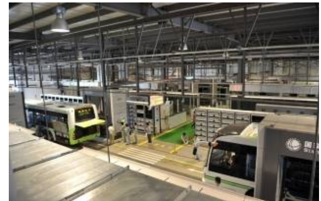
Xuejia Dao EV Battery-swap Station in Qingdao
