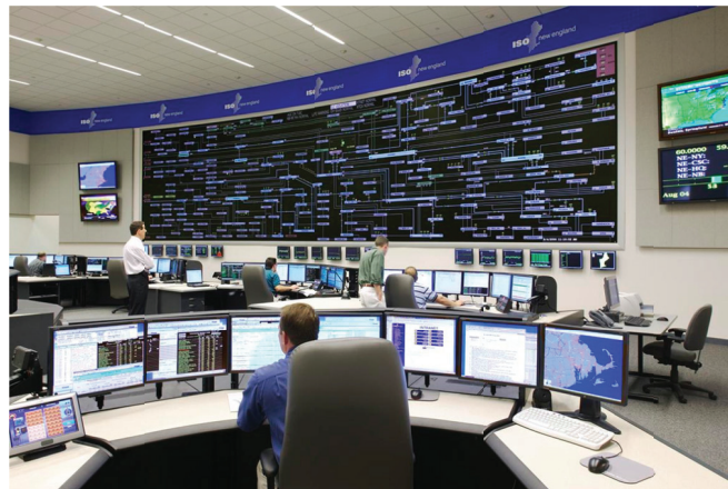
FIGURE 4.7 ISO New England control room. SOURCE: ISONE (2013).
