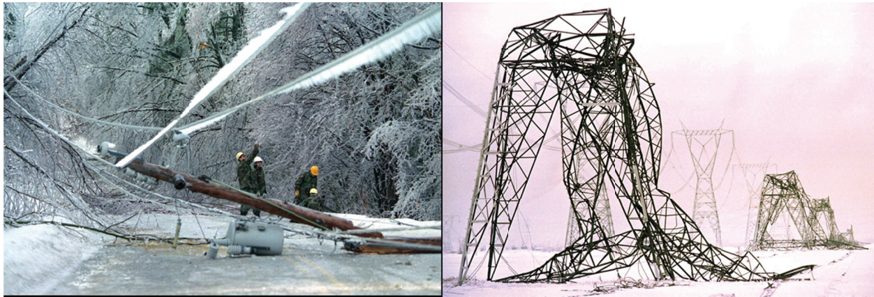
FIGURE 3.10 (A) Ice accumulation of several inches on distribution lines caused these poles to collapse, and (B) images from the infamous 1998 ice storm across southeastern Canada and the northeastern United States. SOURCE: (A) ©1998 The Associated Press (B) Robert Laberge/AFP/Getty Images.
